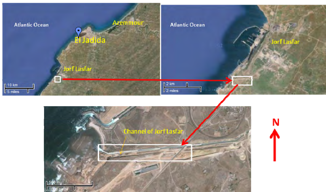
Figure 1. Geographical location of the studied zone (Source of the Photographs: Google Earth).
