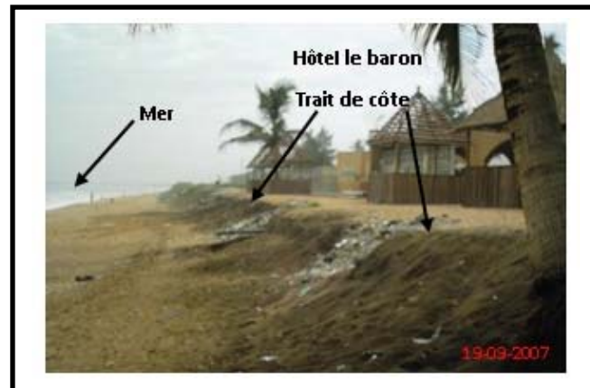
Figure 3. Erosion threat at the level of Hotel Le Baron in Port-Bouët.
