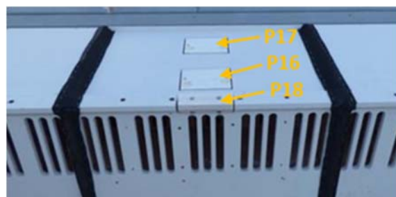
Figure 5. Pressure sensors on roof of caisson n° 3.
