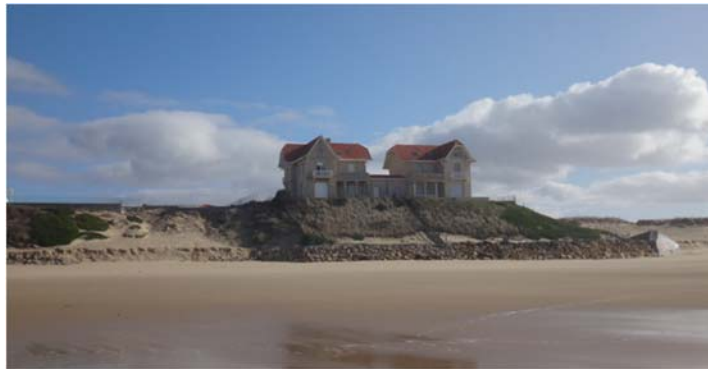
Figure 1. View of the seawall at Biscarrosse Beach at low tide during spring conditions. One can notice the eroded dune front and the side-effect at the seawall on the shoreline retreat.
