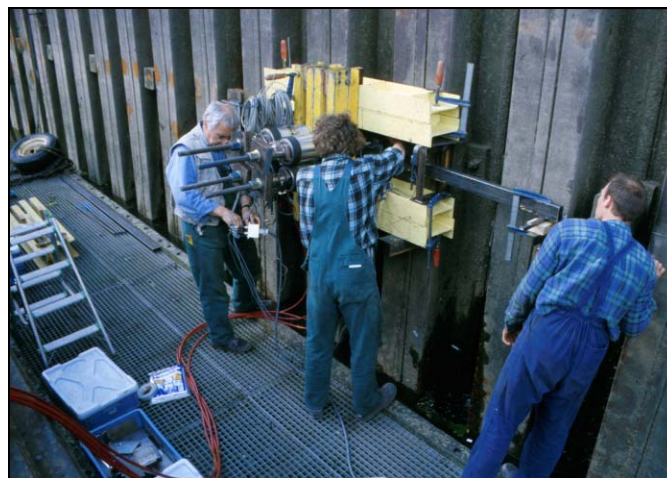
Figure 4. Load tests of anchored sheet pile wall.
