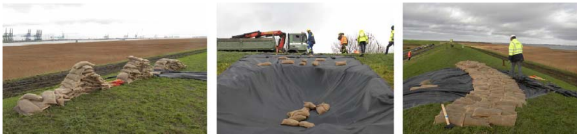
Figure 9. Emergency response to repair the outer slope of a damaged grass covered levee.
