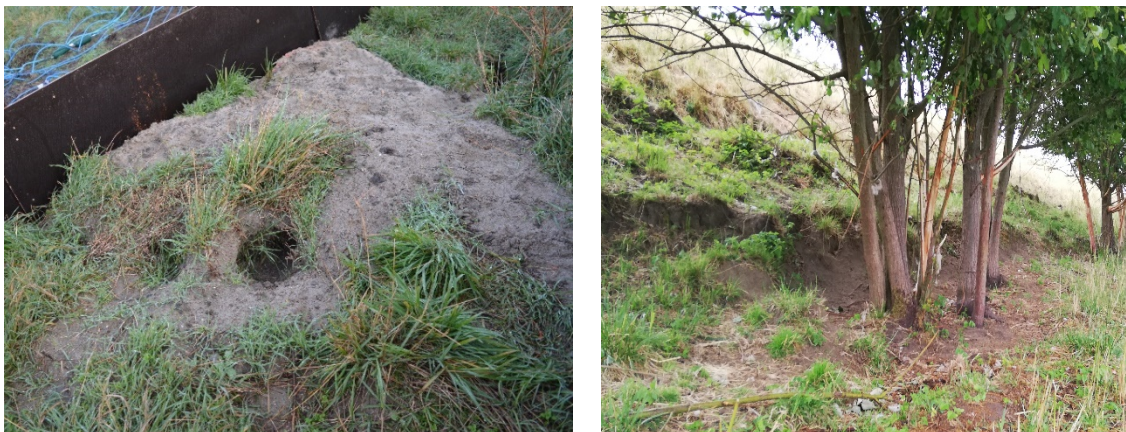
Figure 1. Anomalies being tested under extreme loading conditions: animal burrows (left), (animal-induced) cliffs (right).
