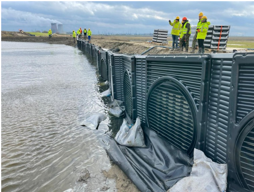
Figure 11. Testing mobile barrier of Cuirassier in Hedwige-Prosperpolder.
