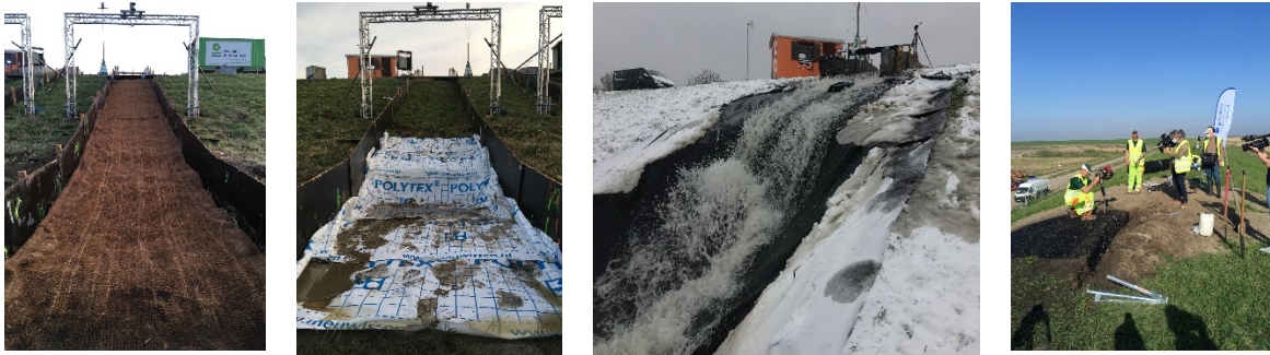
Figure 2. Repairing damage using Cocos mat, Tyvek, EPDM and reinforced turf mat.
