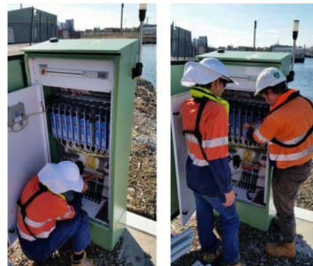
Figure 2. Transformer Rectifier Unit.
