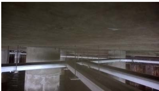
Figure 3. PVC cable tray.
